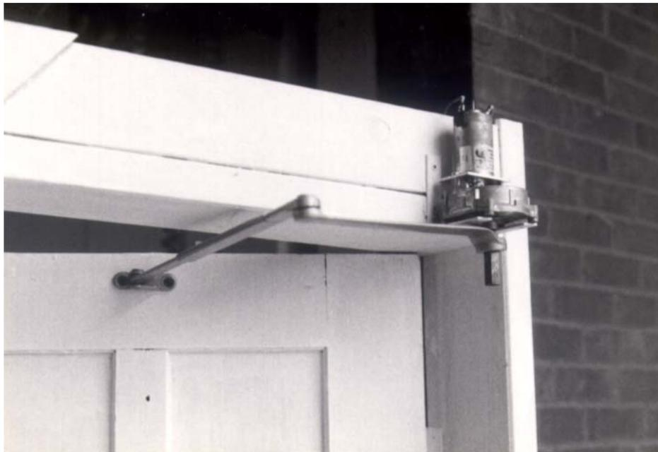
Figure 8.13. 12-volt DC Motor for Door Opener.
