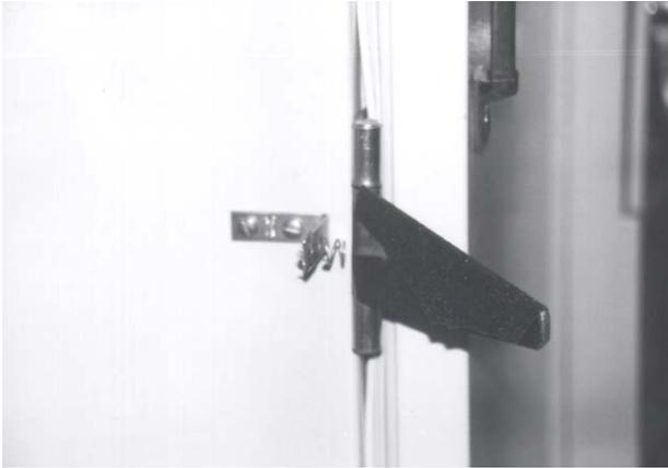
Figure 15.13. Side View Showing Stop Bracket.
