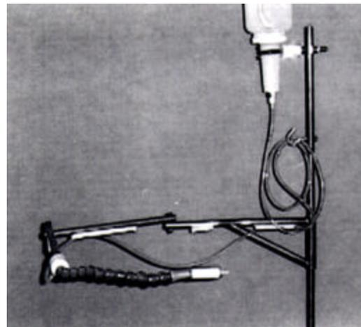
Figure 17.14. Drinking Unit Mounted on a Hospital Bedpost Post with Arm Partially Retracted.
